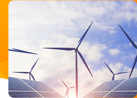
Ground and distributed solar power station
